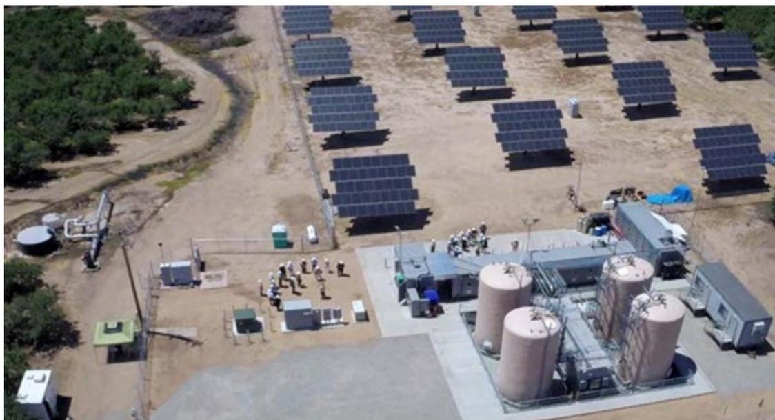
**Figure 3. Photograph of EnerVault Corp.'s 250kW/1MWh Fe-Cr RFB in Turlock, California. Electrolyte is held in the four tanks in the lower right [34].**
