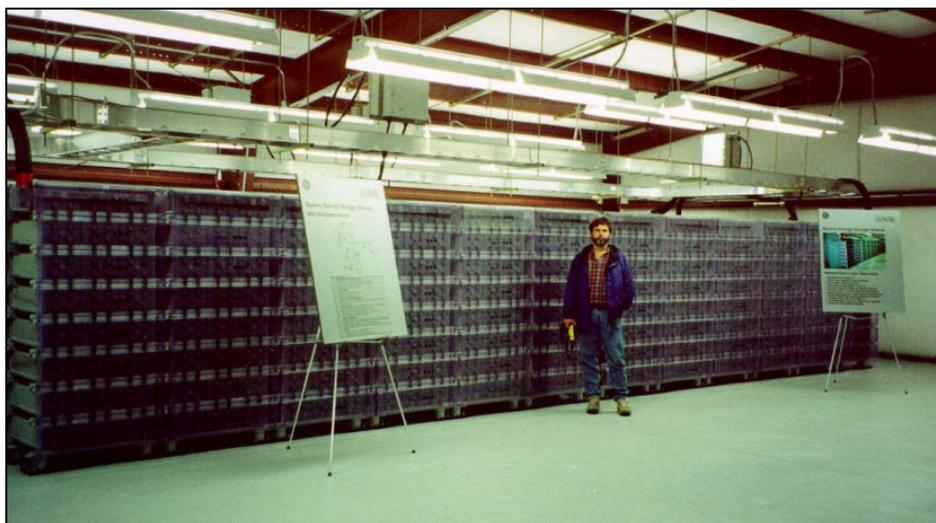
**Figure 70. 1-MW/1.5-MWh Lead-acid Carbon System at Metlakatla, AK<sup>46</sup>**
