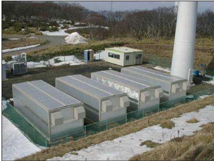
**Figure 71. Acid Battery Installation at Tappi Wind Park**
