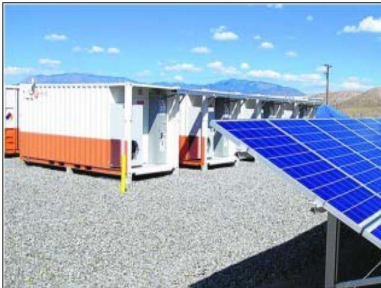
**Figure 73. 500-kW/1-MWh Advanced Lead-acid Battery for Time-shifting and 900-kWh Advanced Carbon Valve-regulated Battery for Photovoltaic Smoothing**
