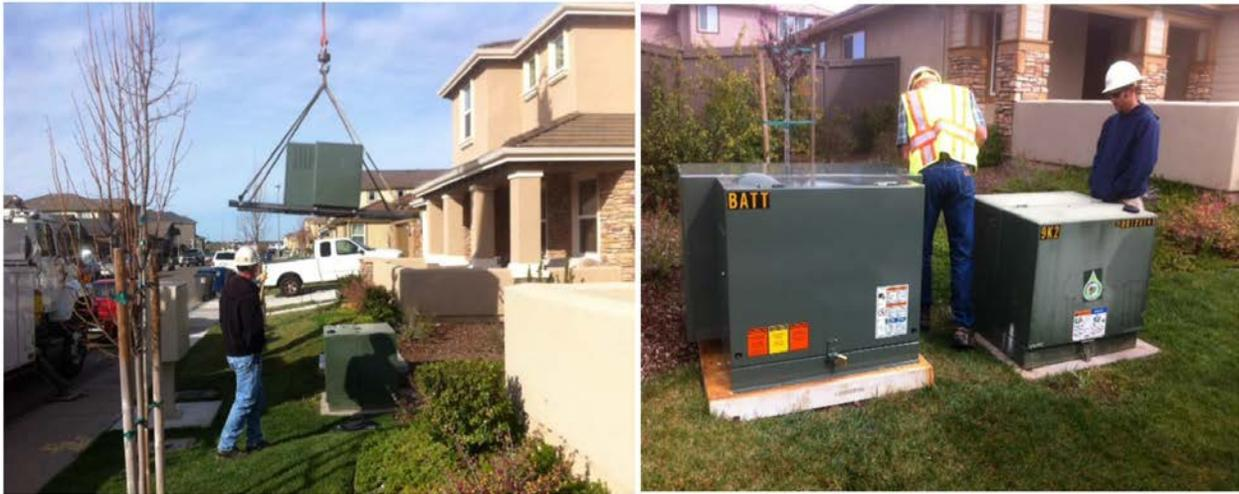
**Figure 99. A 30-kW/34-kWh Distributed Energy Storage Unit**
