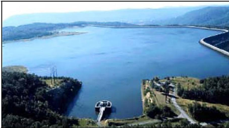
**Figure 21. Man-made Upper Reservoir of TVA's Raccoon Mountain Pumped Hydro Plant**
