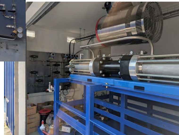
GPS High-Volume Hydrogen Gas Boosting System
