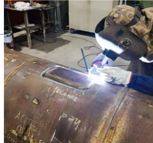
HCF (S-N) Repair N10 weld root
