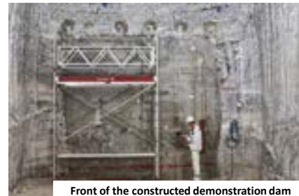
Front of the constructed demonstration dam
