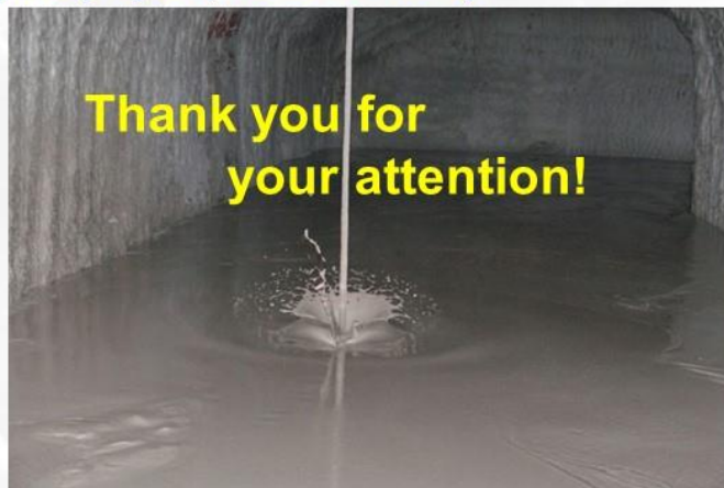
Casting of MgO-Concrete
