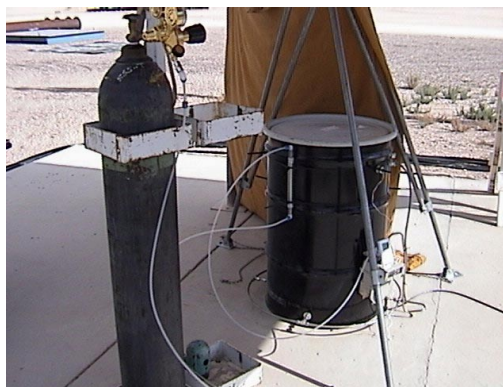
Figure 6. Air-ventilation system connected to the drum.
