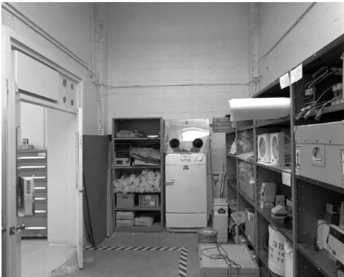
Figure 7. Interior of the center blast wall in Building 904. In 1969, the blast wall was opened, emptied, and turned into two small rooms. This room, 5A, was then used as a centrifuge room, but is currently used for storage. Note the thickness of the wall visible in the doorway. 56
