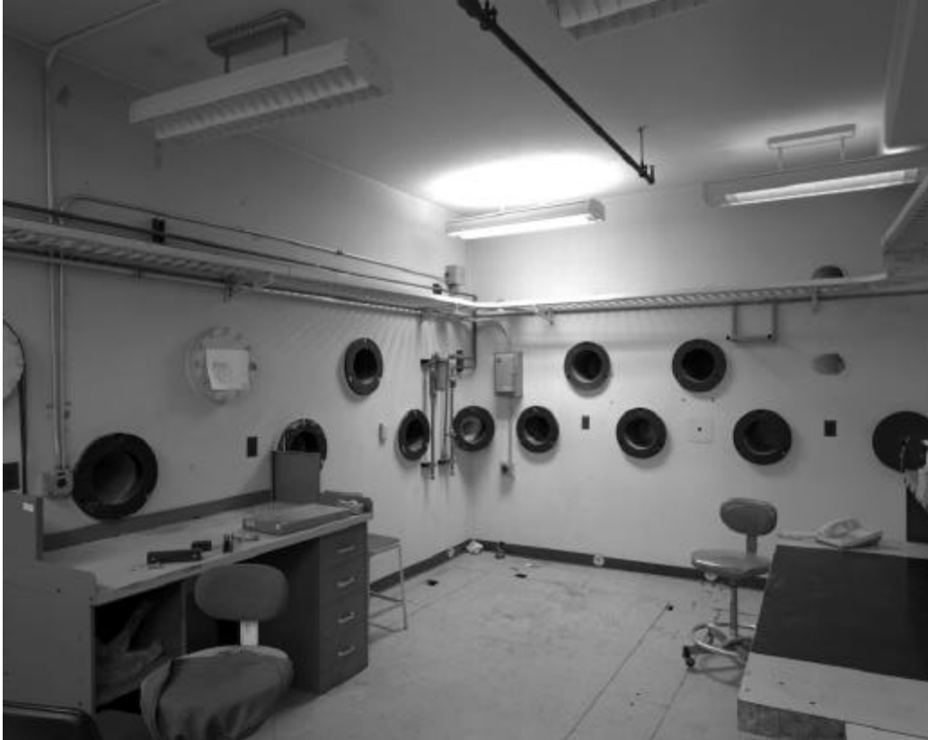
Figure 9. Room 4E in Building 907. Installed as an observation control room in the building in 1962, the room has portholes along its east (left) and south walls. The portholes in the south wall provide a line-of-sight through the various firing pads along the back of the building. 1997 photograph, looking southeast. 82
