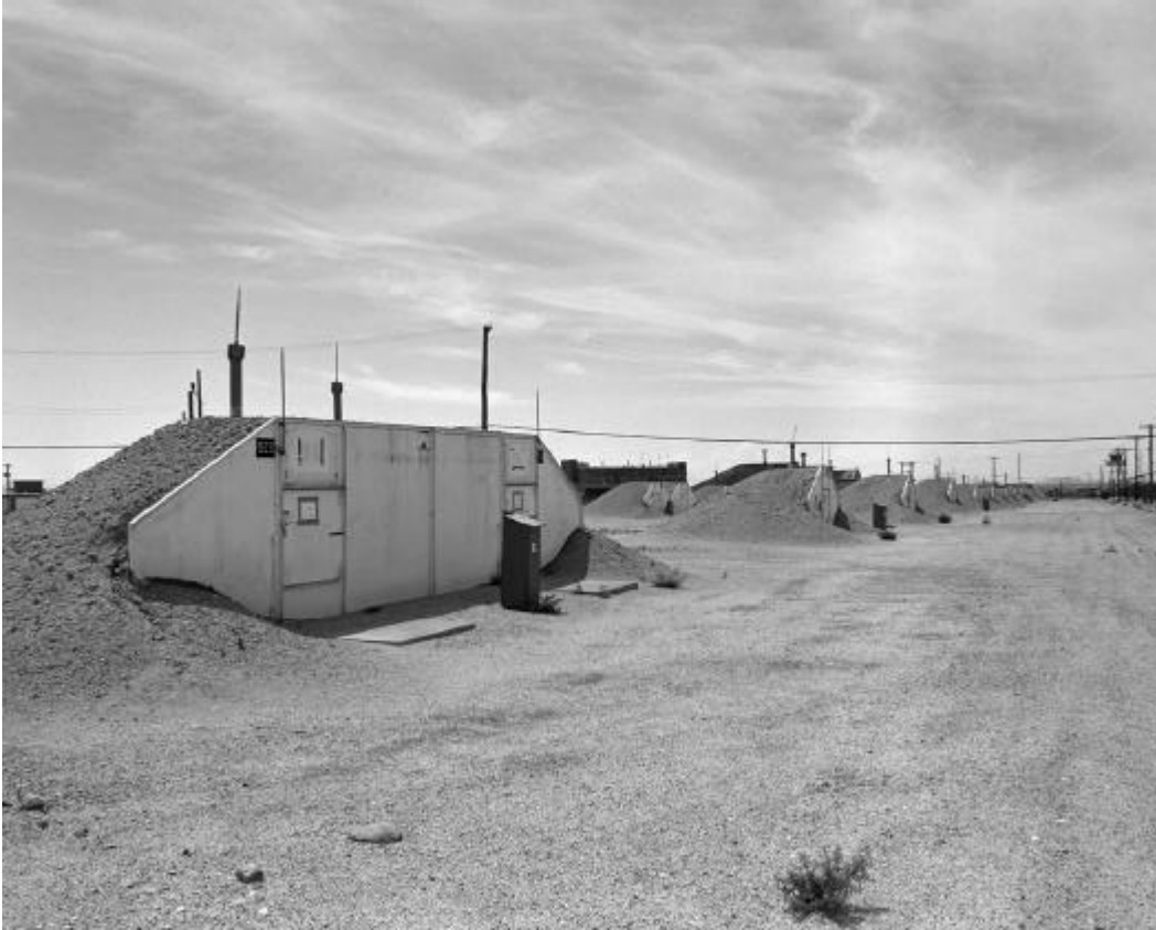
Figure 11. Igloos for storing explosives used in Area II research and testing. This row of igloos faces the northwestern edge of Area II. The dirt blast berms face the rest of the area to prevent propagation should a detonation occur. 84
