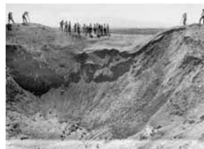
MORE THAN 7,200 tons of earth was tossed out of this 105-foot-diameter crater created by the detonation of a buried charge of 30,500 pounds of high explosives.
