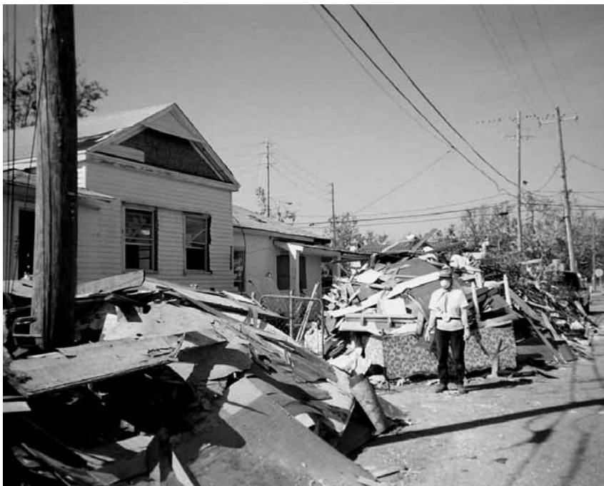
THIS WAS A SCENE volunteers confronted as they began the flood clean-up and started helping in the rebuilding process.
