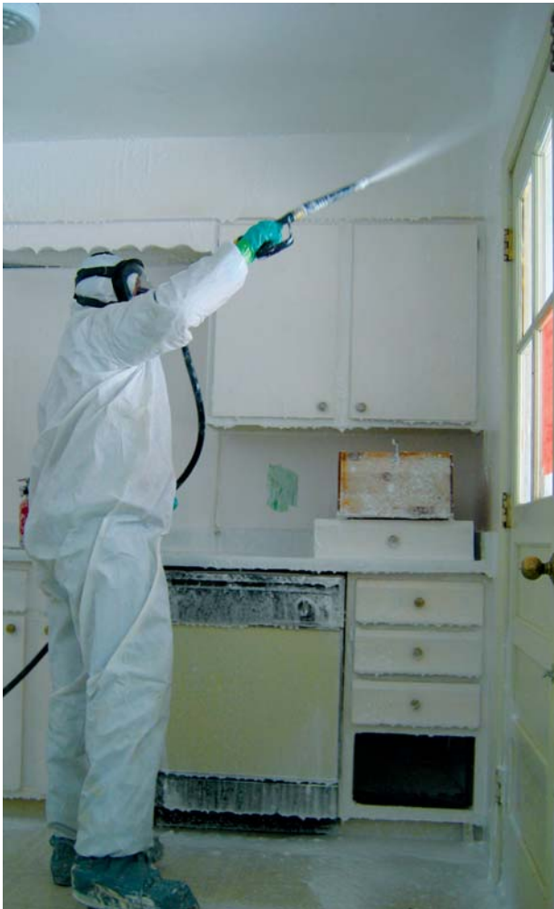
A REMEDIATOR sprays Crystal Clean on surfaces of a house contaminated with methamphetamine. In an hour, the foam is rinsed clean with water, and the remaining liquids are harmless enough to be put down a kitchen drain. (Photo courtesy of EFT Holdings)
