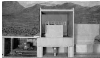
THE SANDIA ENGINEERING REACTOR FACILITY (SERF) shown in this cutaway model reveals the remote handling facilities used to transport test materials in and out of the radiation cell (center).
