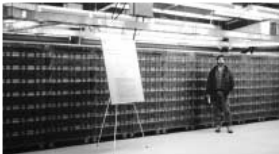
METLAKATLA BATTERY ENERGY STORAGE — Nick Miller of General Electric, who served as technical manager of the Metlakatla, Alaska, battery energy storage project, is in the battery room. The picture was taken in August 1997 when the system was dedicated.
