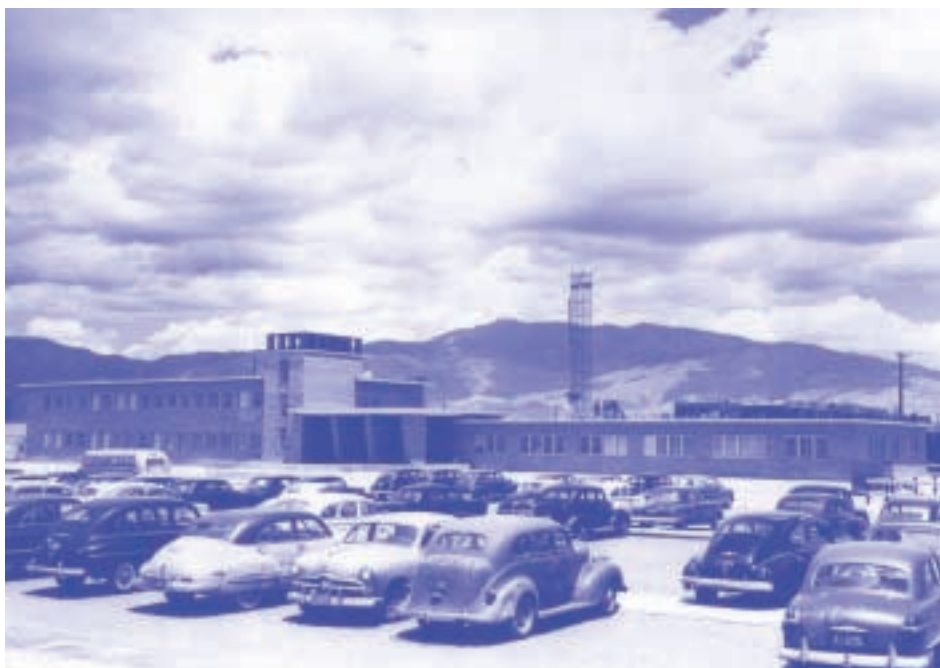
BLDG. 800 WHEN IT WAS NEW — This photograph shows Bldg. 800, Sandia's "front door," as it looked when it was completed 52 years ago.
