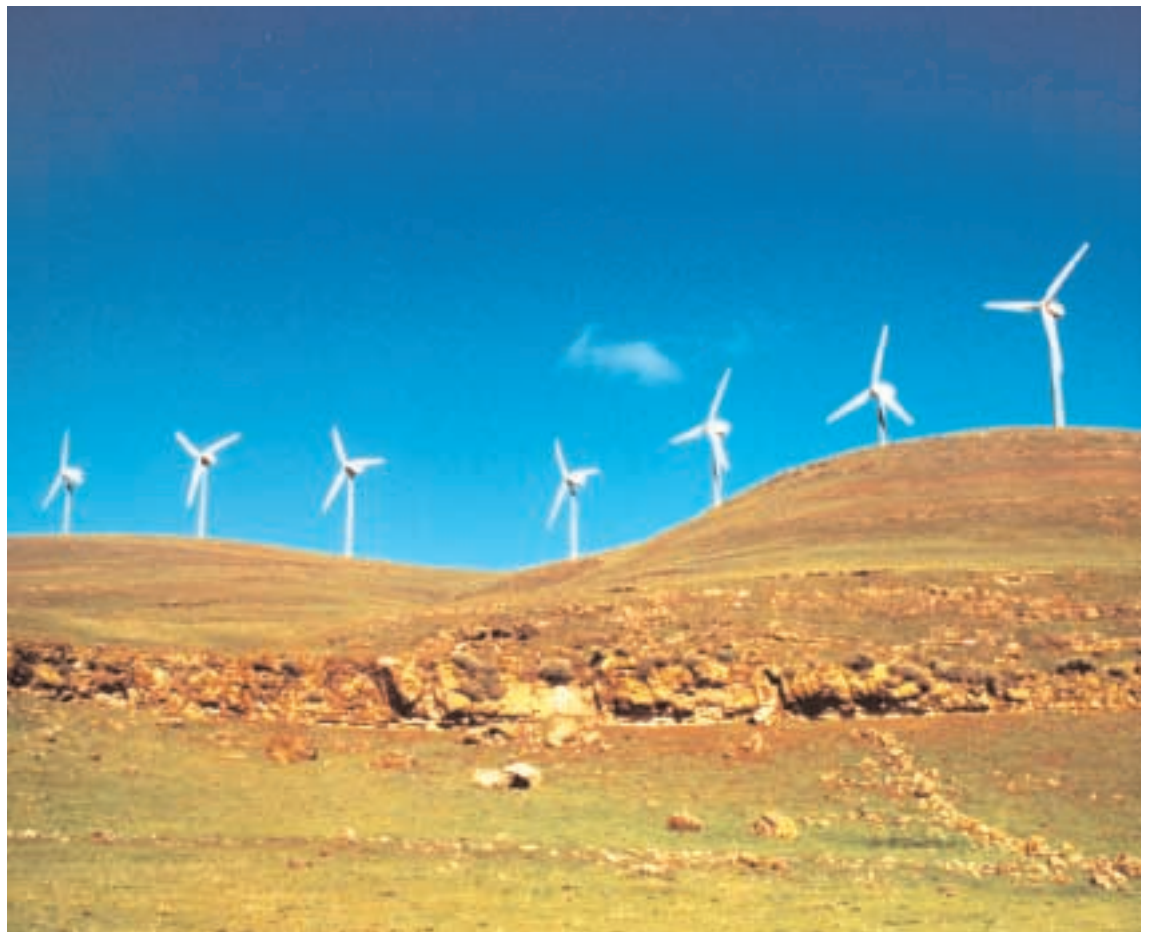
WIND FARM — Windmills dotting the scenic Altamont Pass behind Livermore are electric turbines that were designed to produce alternative energy. (Photo by Lynda Hadley)
