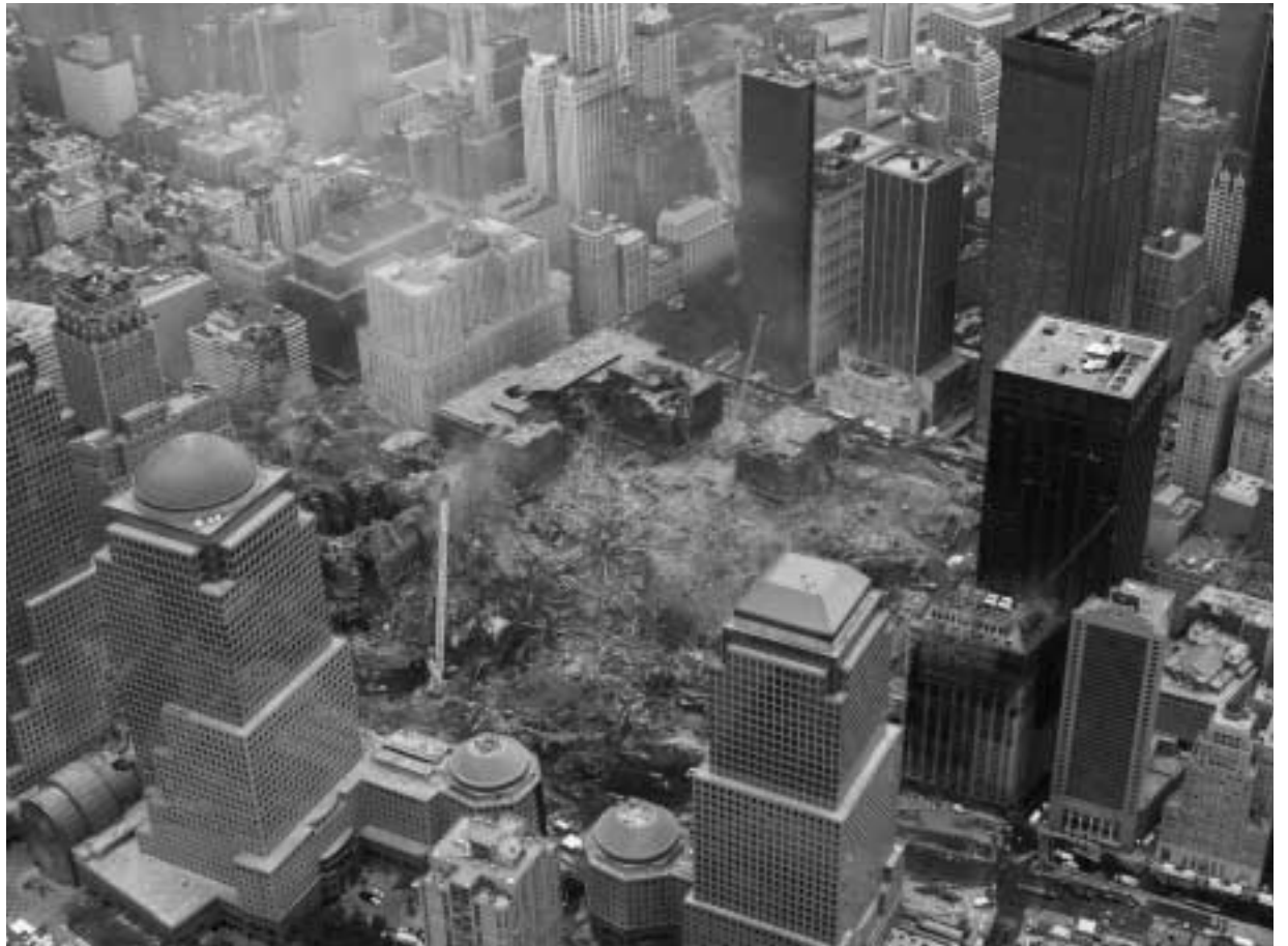
RESEARCHERS from all over Sandia have contributed much to the Labs' ability to answer the nation's call following Sept. 11 with regards to the vulnerabilities of structures to attacks. (Photo courtesy of FEMA)
