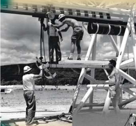
Sandia field testers for Operation Dominic installed a Nike booster on a launcher at Kauai in May 1962.
