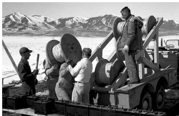
LOADING A CABLE TRAILER, 1950s. Atomic tests used lots of cable.
